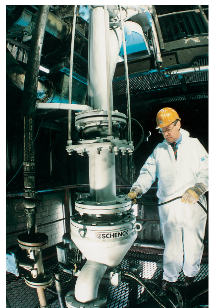
STENFLEX® type R-1 in a proportioning system
