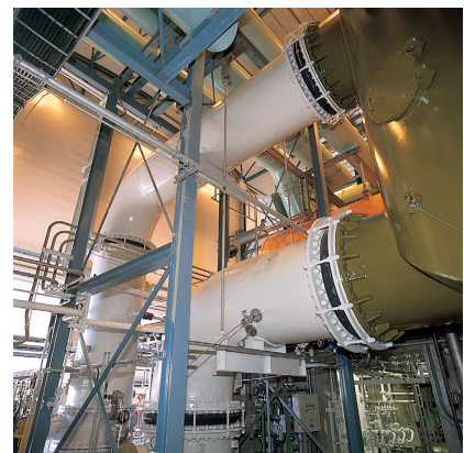
STENFLEX® type C-31 in a power plant
