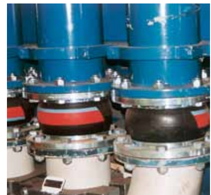
STENFLEX® type AS-1 used in cooling water system of ship's engine
