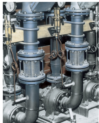
STENFLEX® type SR-2 at pumps
